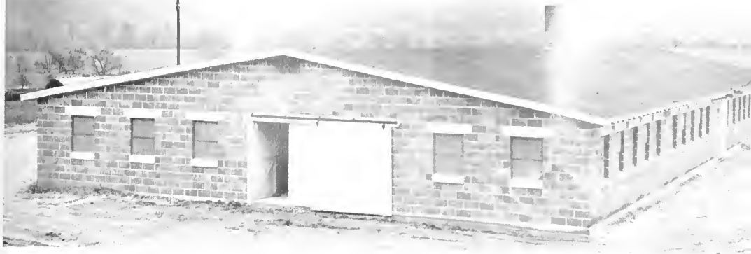
BROILER HOUSE, REYMANN MEMORIAL FARMS, HEATED WITH HOT AIR FROM CENTRAL LOCATION.
